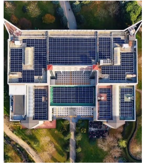
Figure 3. Solar panel installation at Okan University. Okan university Instagram
