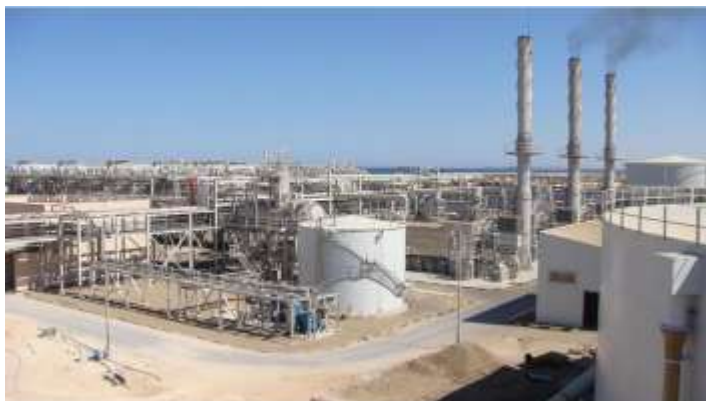
Figure 35: Air pollution at Zwara Desalination Plant.
