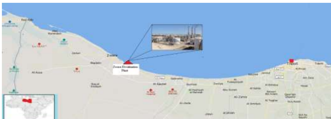
Figure1: Location of the Zwara Desalination Plant on the Libyan Coastline
